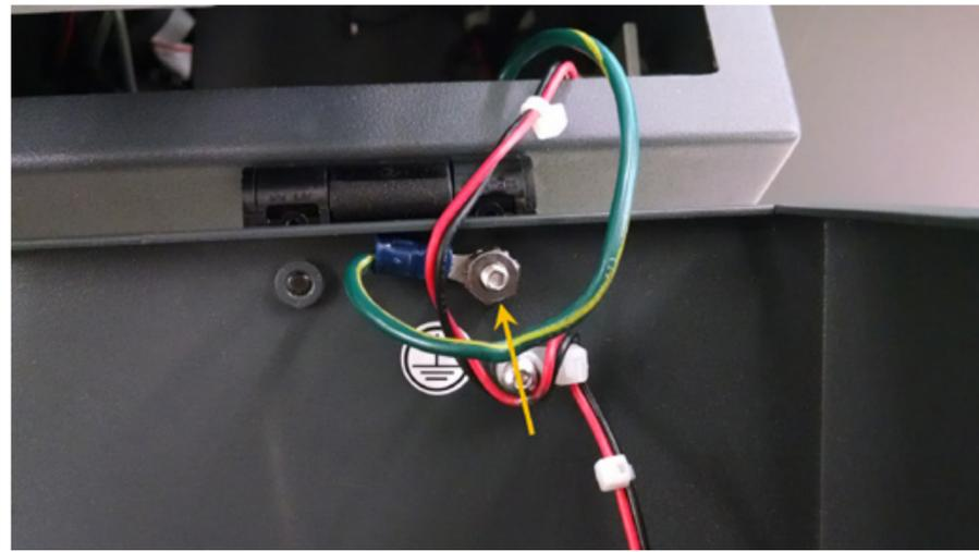
5. Remove the screw holding the wire tie that secures the exhaust fan power cable.
