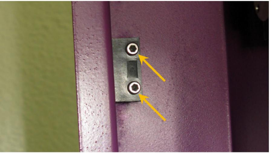
4. Installation is opposite of removal. Ensure the magnet is flush with the top door frame or slightly sticking out.
